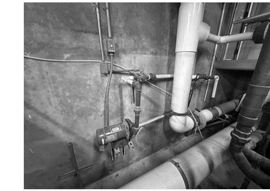
8 Circulator Piping Behind Boiler M100 NTS
