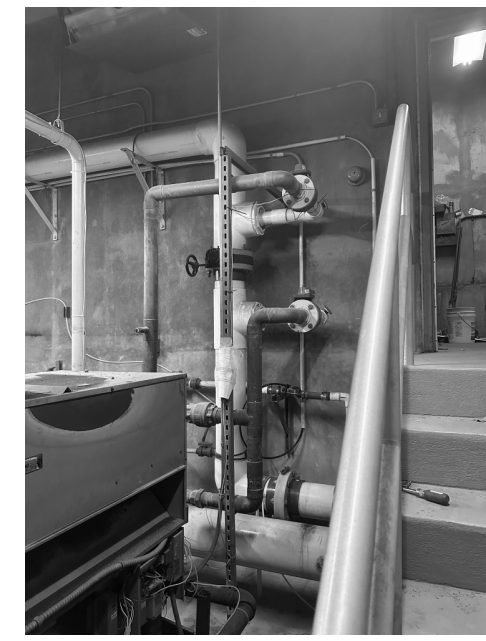
5 Heater Circ Piping M100 NTS
