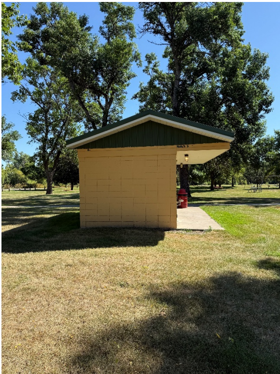
West Side of Building
