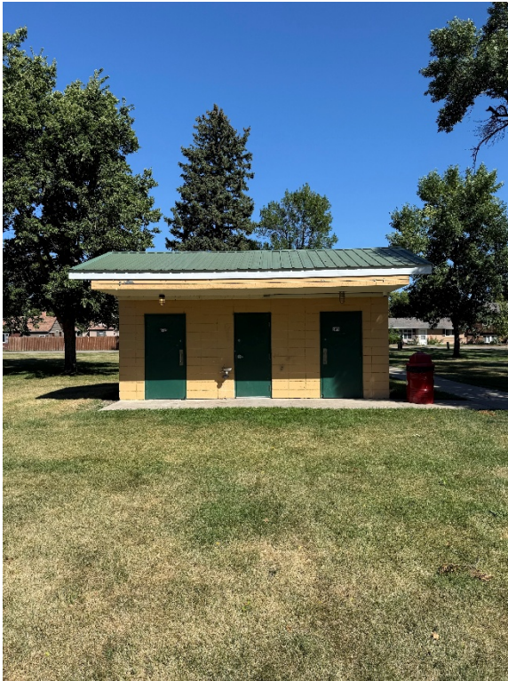
South Side of Building
