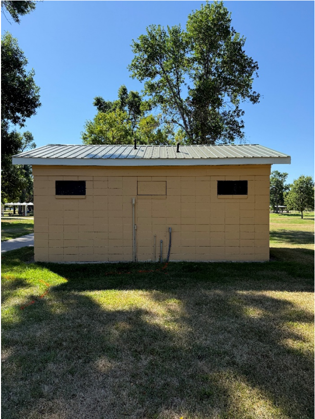
North Side of Building
