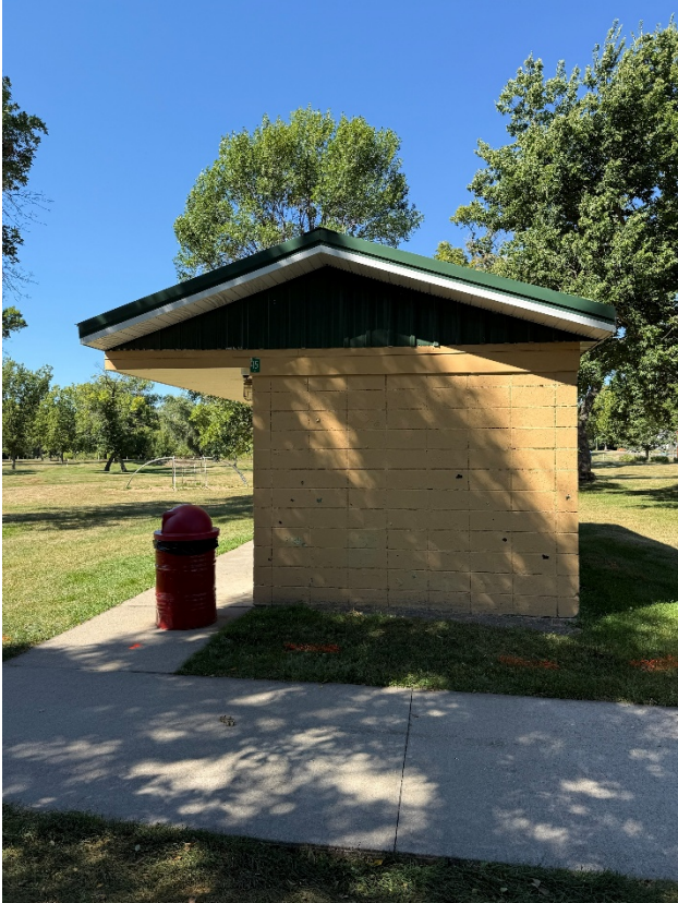
East Side of Building
