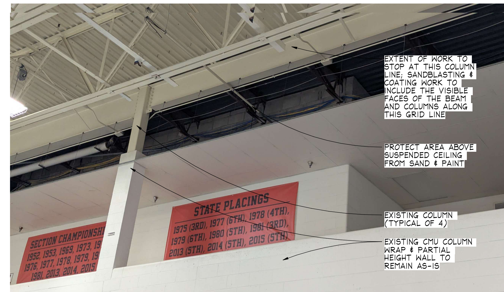
IMAGE 3 EAST INTERIOR WALL & COLUMN LINE (LOOKING EAST)
