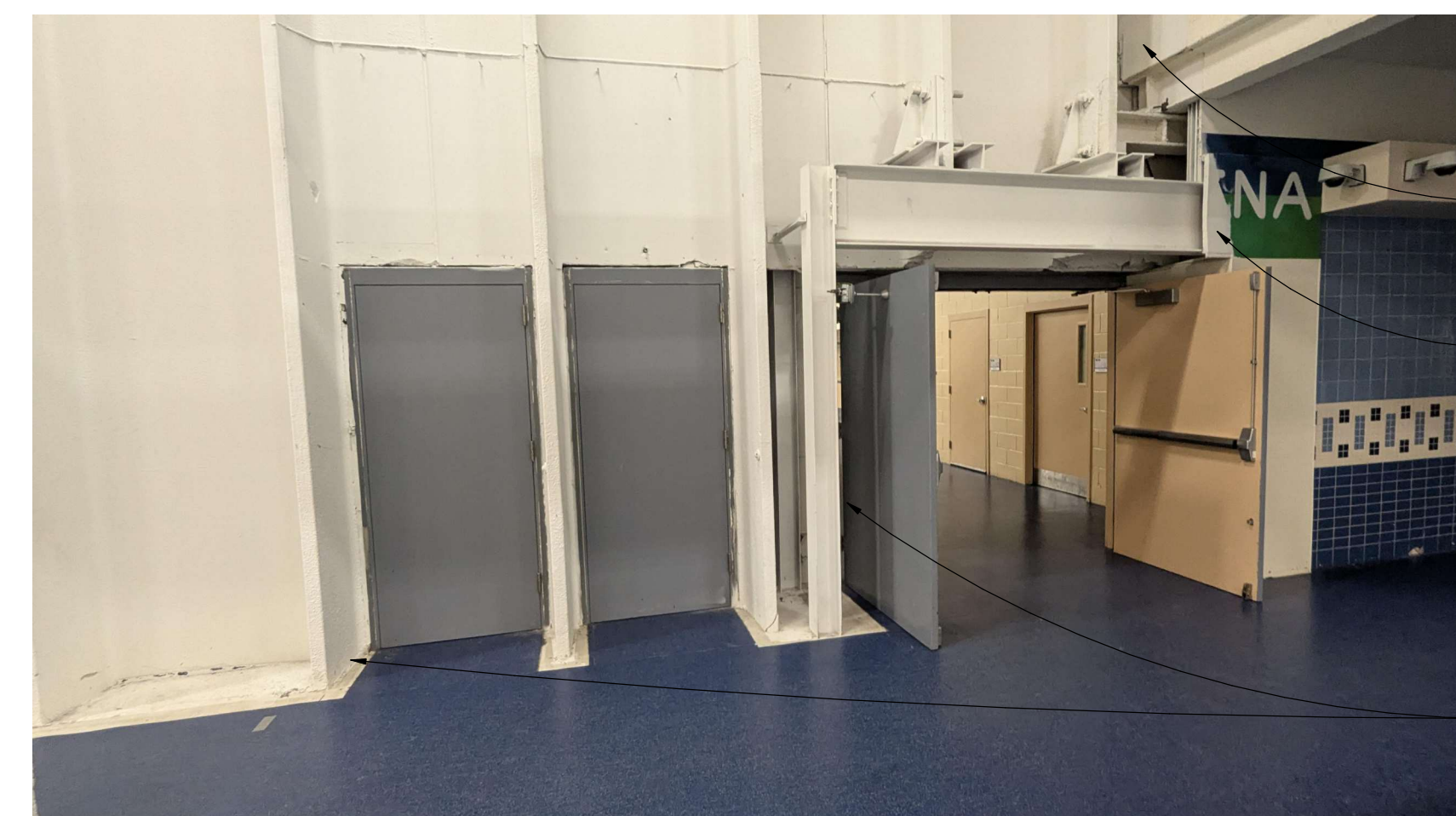
IMAGE 4 SOUTHWEST WALL AT DOOR ALCOVE (LOOKING SOUTH)
